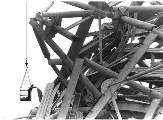
**Figure 29-1** The football stadium add-on at the University of Washington collapsed because it wasn't strong enough to support itself during construction. It likely would have been strong enough when completed, but it was constructed in the wrong order—an integration error.
