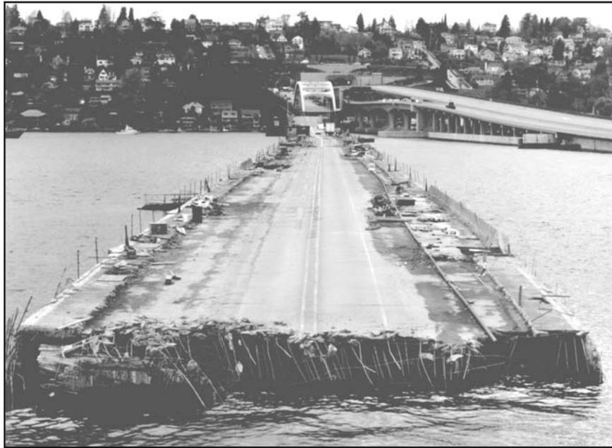
**Figure 8-1** Part of the Interstate-90 floating bridge in Seattle sank during a storm because the flotation tanks were left uncovered, they filled with water, and the bridge became too heavy to float. During construction, protecting yourself against the small stuff matters more than you might think.
